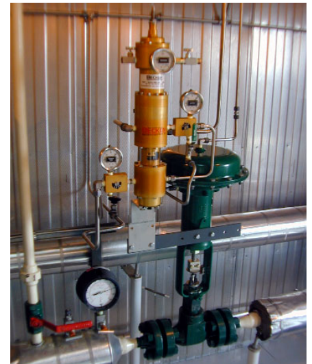
Figure 9.0 - VRP-SB-CH Retrofit Virtually Eliminates Atmospheric Bleed Gas
