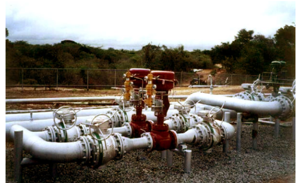
Figure 10.0 – Becker model VRP-175-SB-CH single-acting pilots installed on Masoneilan globe valves with spring & diaphragm actuators (above) and spring & piston actuators (below). Installations are in South America.
